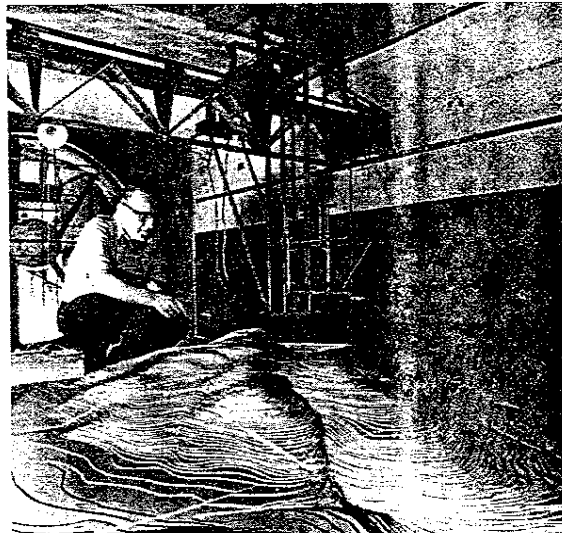
In a Technion wind tunnel, Prof. Michael Poreh studies a model of the Yodfat ridge, proposed site of a 20-MW wind farm.
